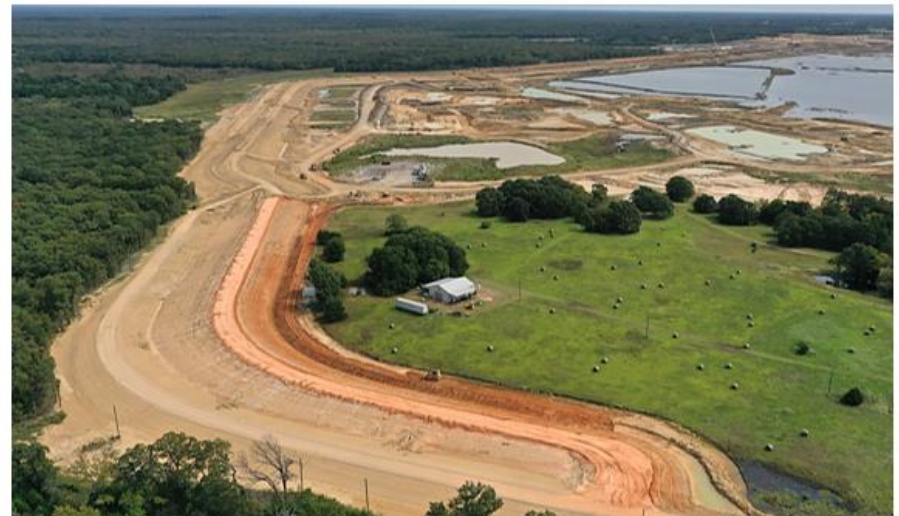
CMAR 1 – Archer Western – CR 2700 re-align and west dam embankment.
