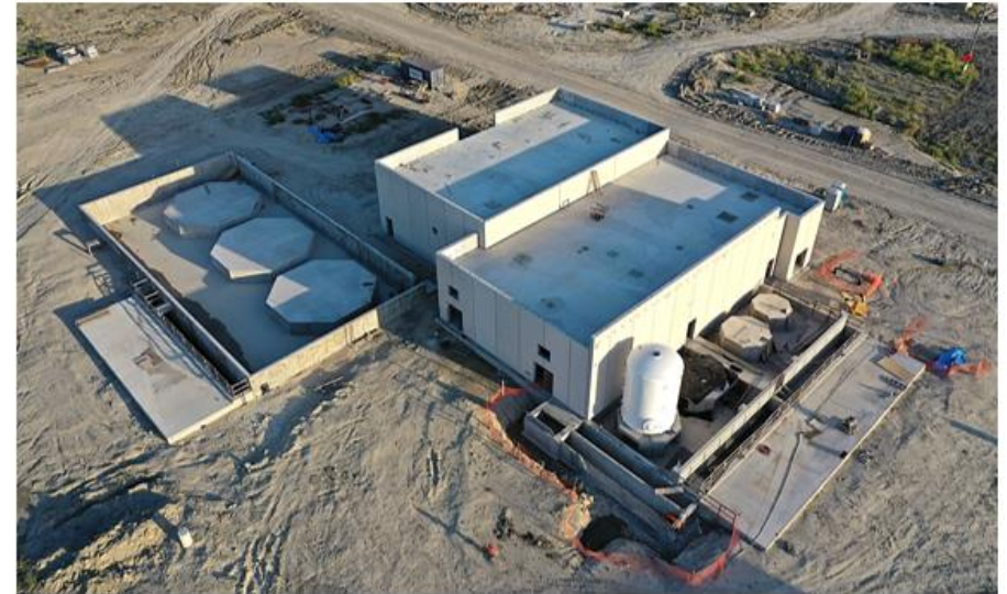
CMAR 3 – Garney – LWTP north chemical storage building.
