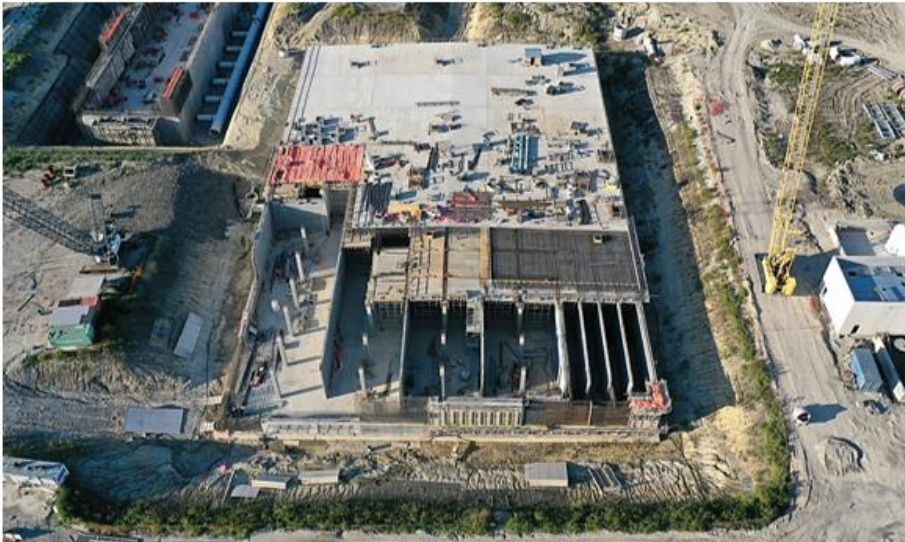
CMAR 3 – Garney – LWTP chlorine contact basin and clearwells.
