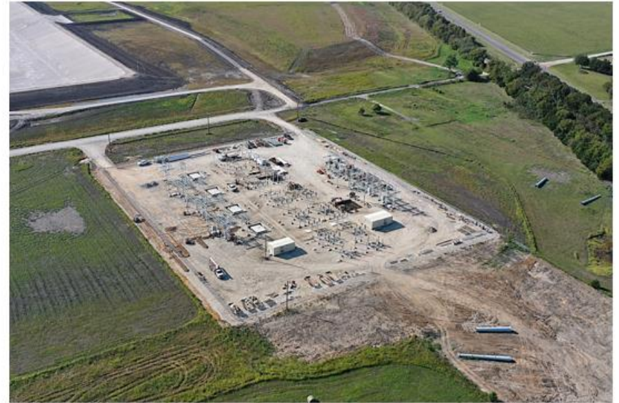
CMAR 1 – Archer Western – TSR nearby substation construction.
