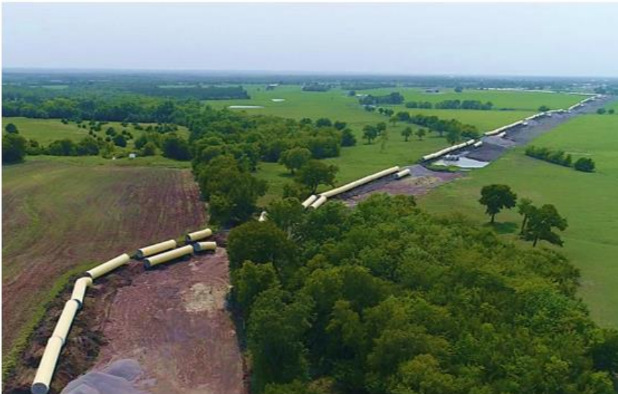
CMAR 5 – Garney – TWPL Segment D pipe staging.
