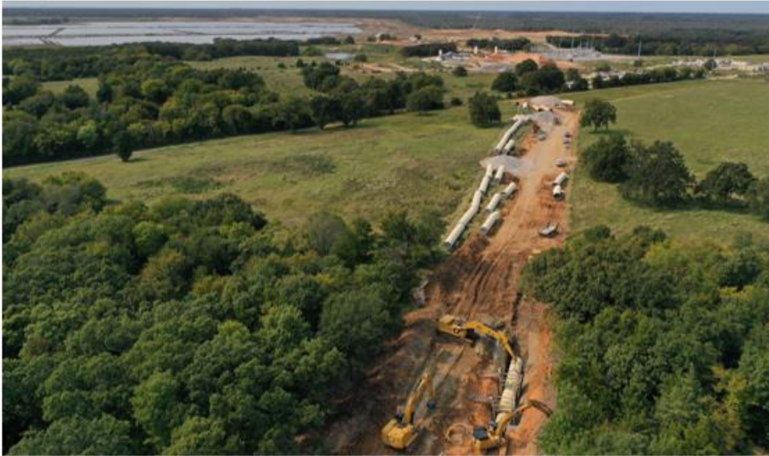
CMAR 5 – Garney – RWPL Segment A approaching the outfall pipe.
