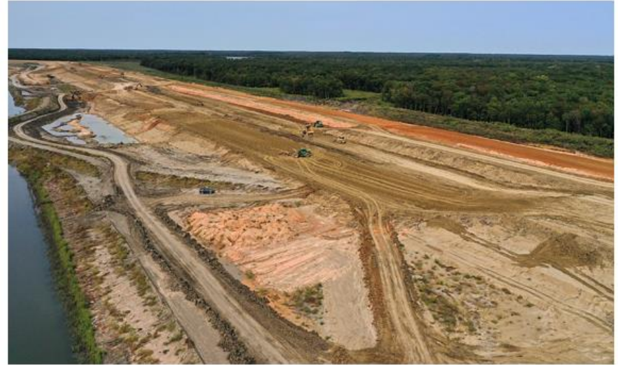
CMAR 1 – Archer Western – Embankment work on the notch closure.
