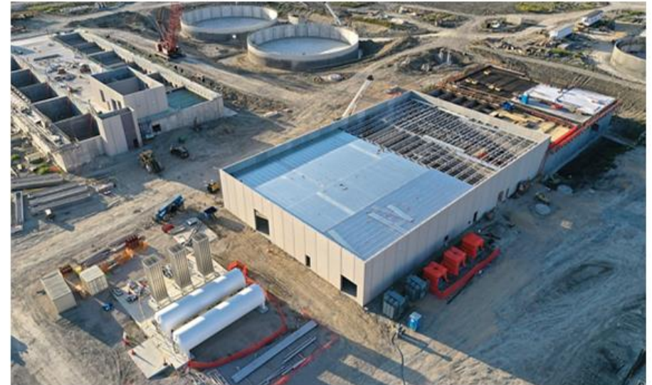
CMAR 3 – Garney – LWTP ozone structure.
