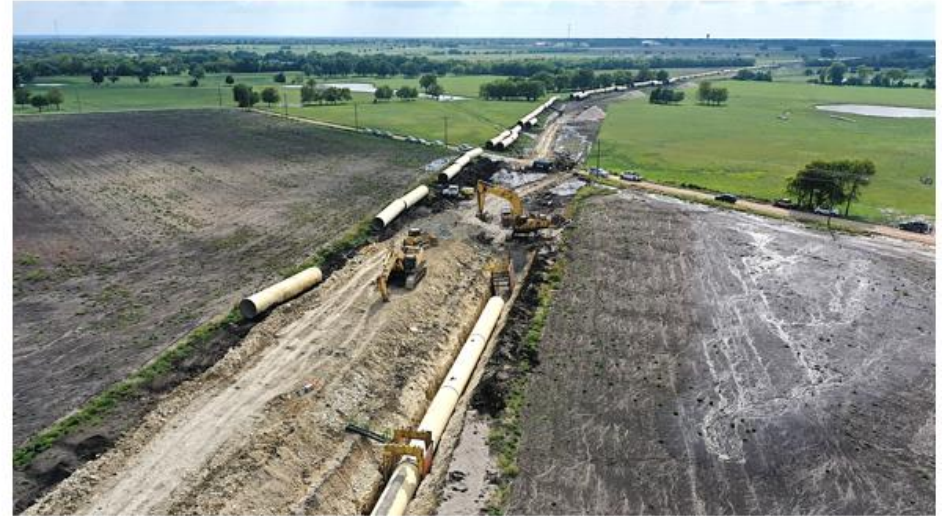
CMAR 5 – Garney – RWPL Segment C installation near CR 4830 .
