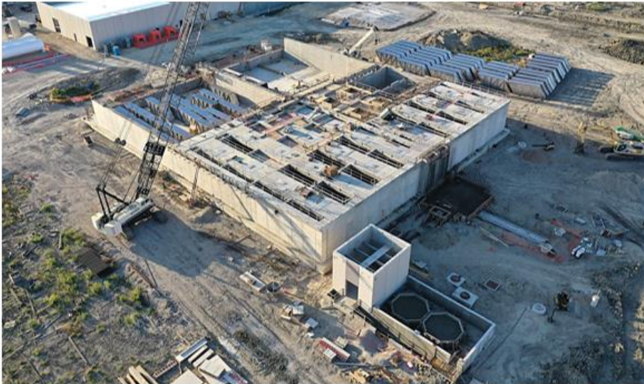
CMAR 3 – Garney - LWTP pre-treatment building.
