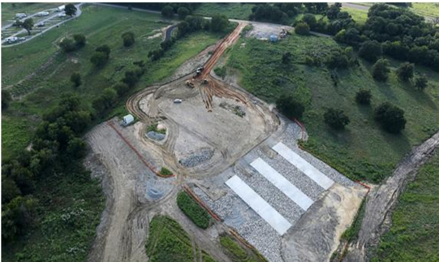
CMAR 4 – Austin Bridge and Road – FM 897 boat ramp aerial view.
