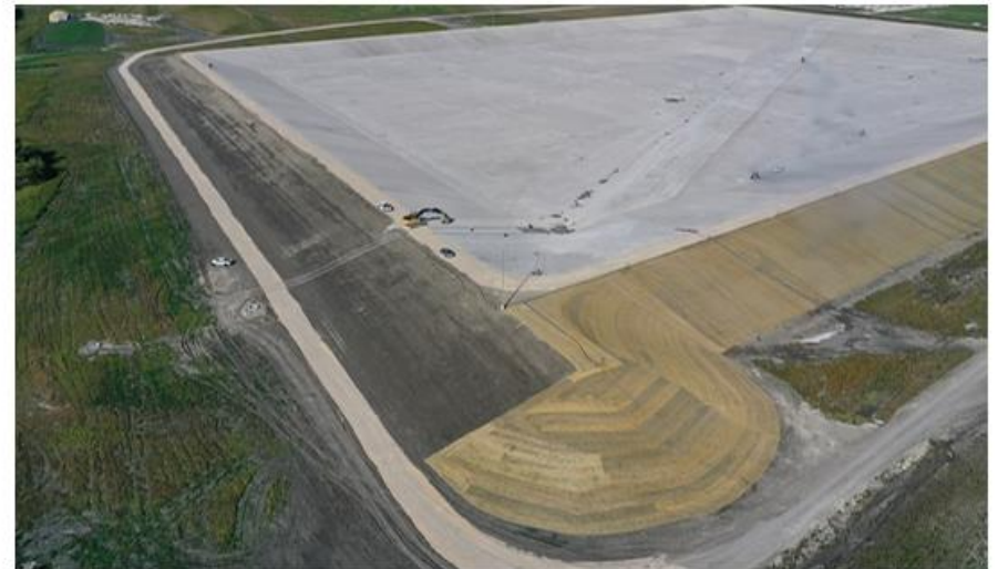
CMAR 1 – Archer Western – TSR seeding and sodding the south slope of embankment.
