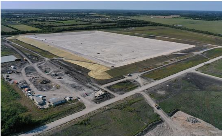
CMAR 1 – Archer Western – TSR aerial looking northwest.
