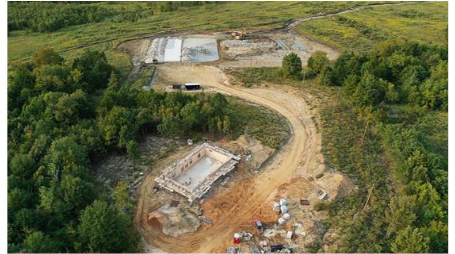
CMAR 4 – Austin Bridge and Road – Construction on the bunkhouse and private boat ramp.
