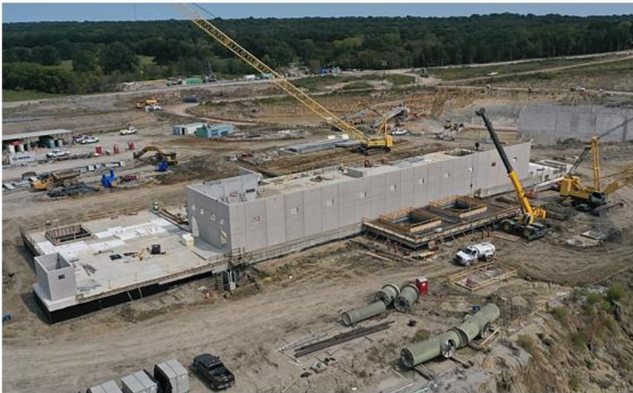
CMAR 3 – Garney – RWPS precast wall installation.
