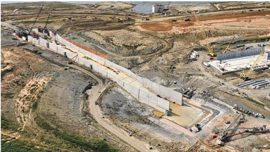
CMAR 1 – Archer Western – Service spillway stilling basin soil cement activity.
