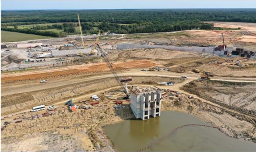
CMAR 1 – Archer Western – Intake tower aerial view.
