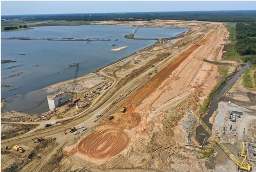
CMAR 1 – Archer Western – Aerial of dam embankment looking west.
