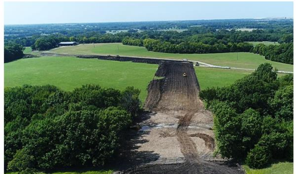
CMAR 5 – Garney – TWPL Segment E ROW stripping activities.
