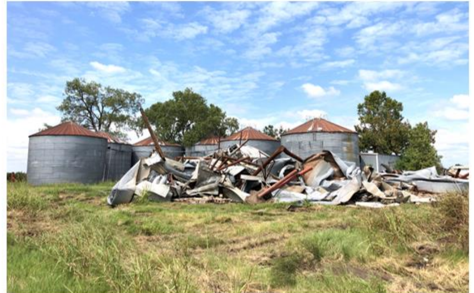
Mitigation FSP – RES – Demolition of grain silos.
