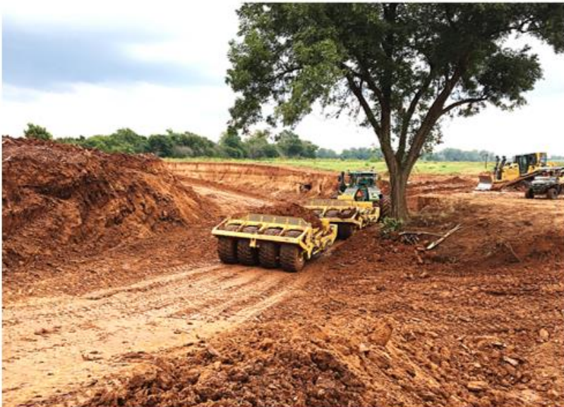
Mitigation FSP – RES – Willow Branch main plug reconstruction.
