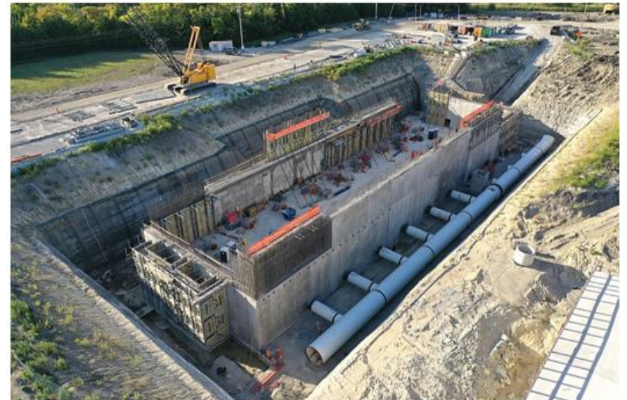
CMAR 3 – Garney – HSPS forming, reinforcing, and placement of walls.
