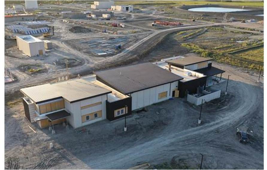
CMAR 3 – Garney – LWTP operations building.
